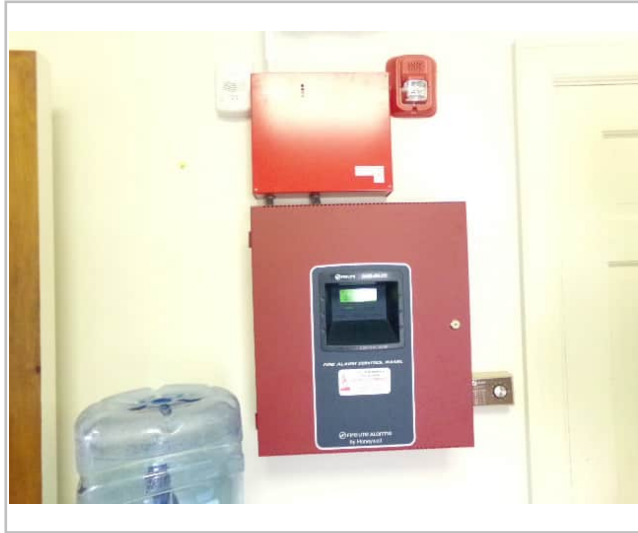
SUBJECT PROPERTY INTERIOR
