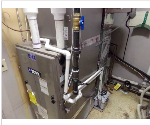
SUBJECT PROPERTY INTERIOR
