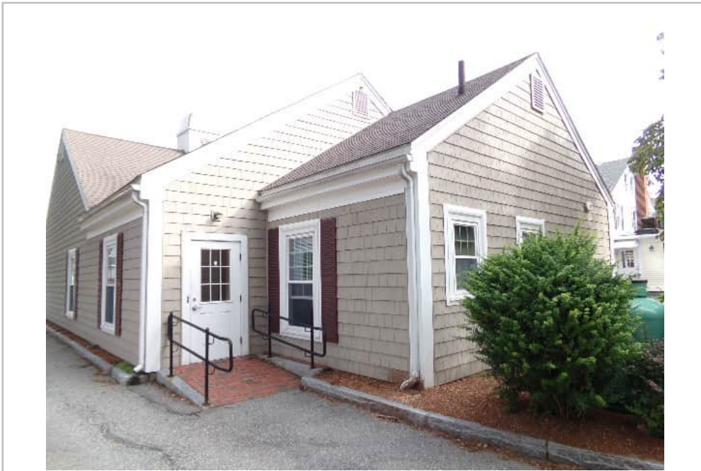
SUBJECT PROPERTY REAR VIEW
